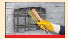
Clean reinforcement steel with a wire brush.
