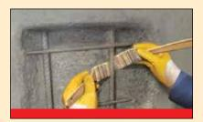
Apply corrosion inhibitor to clean the damaged rod.
