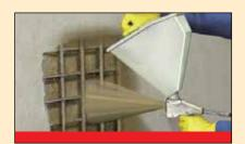
Pour the mixed Ramco Micro Concrete immediately. Avoid vibration or compaction, ensuring a continuous pour.
