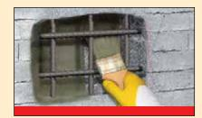
Apply Ramco Super Bond Epoxy to steel and old concrete
