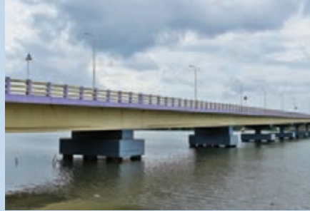
Thevara Bridge (Kerala)
