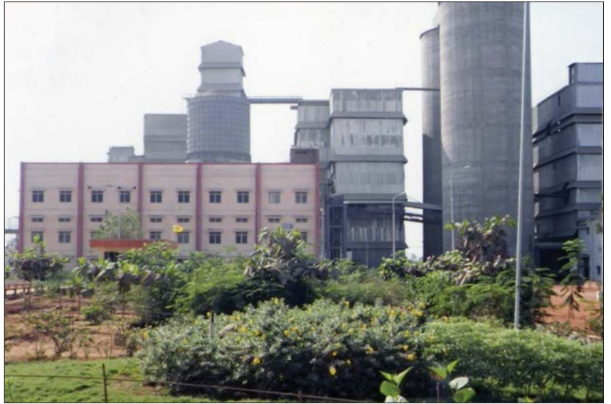
A view of the Chengalpattu Grinding Plant.
