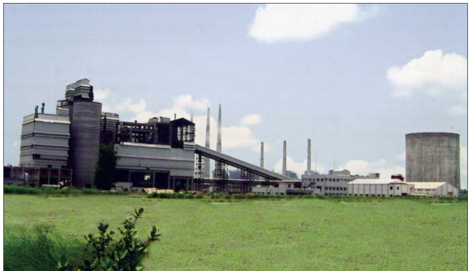
A view of the Kolaghat Grinding Plant.
